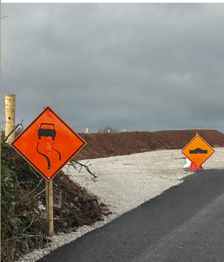
Passing bays installed to reduce road closures.
