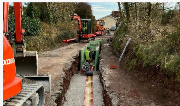
Trenching and ducting works progressing.
